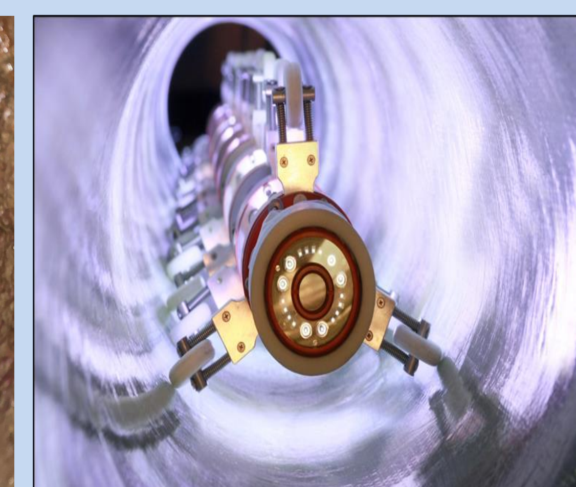
Cure liner to bond to host pipe
