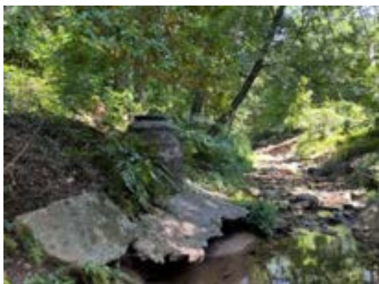
Exposed sanitary sewer manhole with undercut concrete base, indicating potential structural vulnerability
