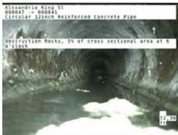
Sediment and rock obstructions and discoloration of pipe lining.
