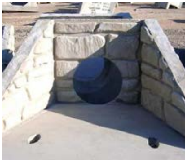
Example of rock façade finish for outfalls
