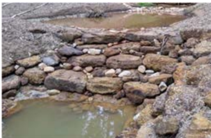
Example of boulder cascade following Regenerative Step Pool Conveyance Design Guidelines
