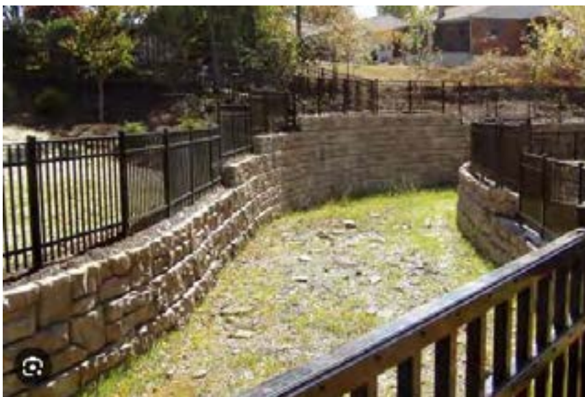
Example of gravity retaining wall with safety railing
