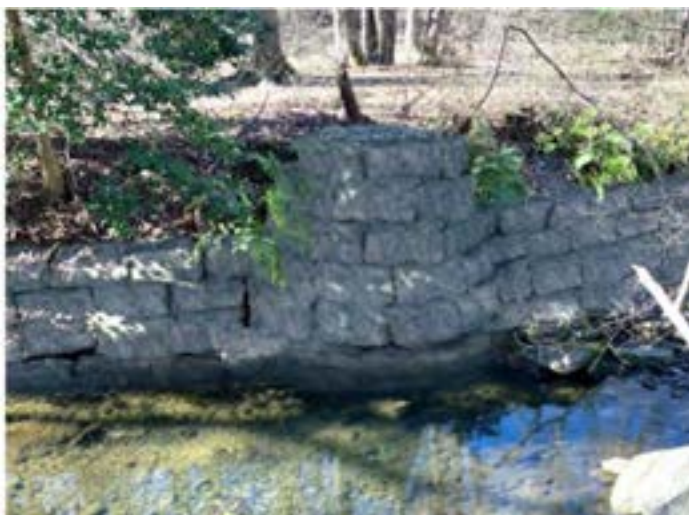
Example of sanitary sewer manhole protection
