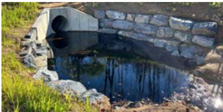
Example of plunge pool downstream of outfall
