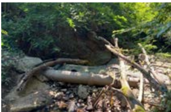
Exposed sanitary sewer line vulnerable to erosion and structural damage
