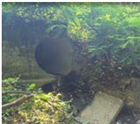
36-inch stormwater outfall showing significant undercutting and headwall deterioration
