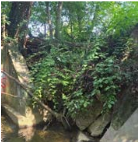
Erosion observed behind the right wingwall of the outfall (viewed looking upstream)
