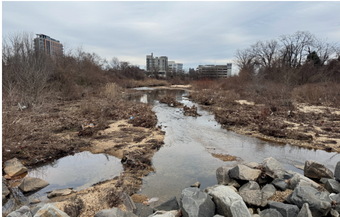
Sedimentation downstream of Weir #1
