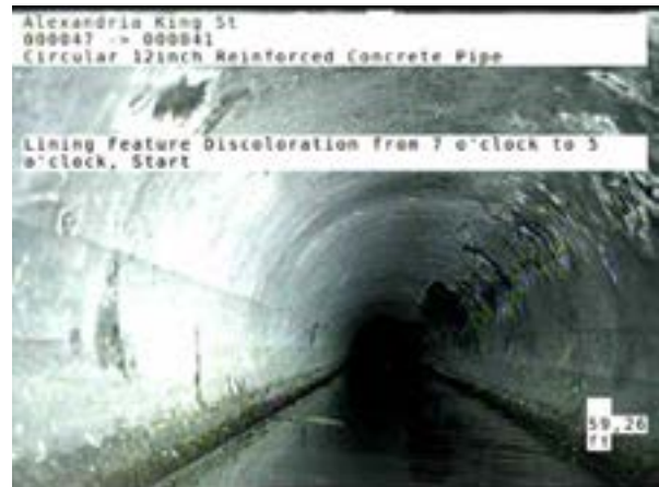
6, 00:04:39, 59.26ft Lining Feature Discoloration from 7 o'clock to 5 o'clock, Start
