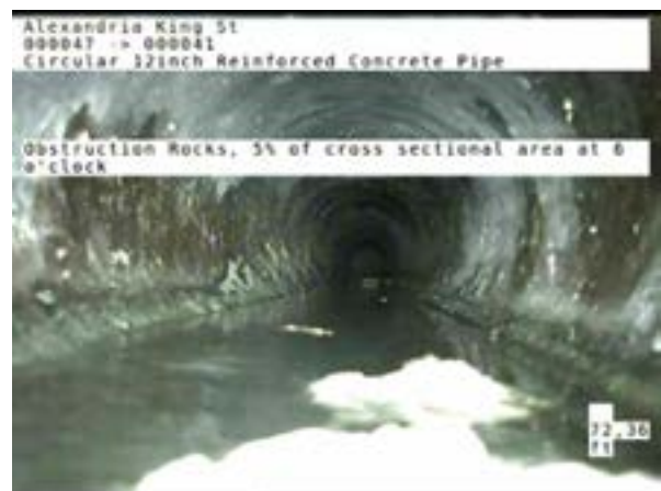
8, 00:05:38, 72.36ft Obstruction Rocks, 5% of cross sectional area at 6 o'clock
