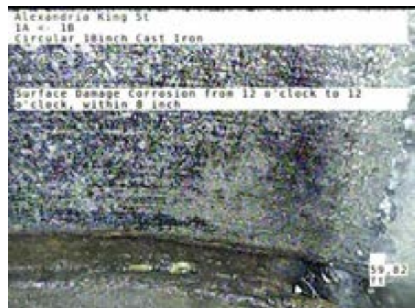
4, 00:03:32, 59.82ft Surface Damage Corrosion from 12 o'clock to 12 o'clock, within 8 inch
