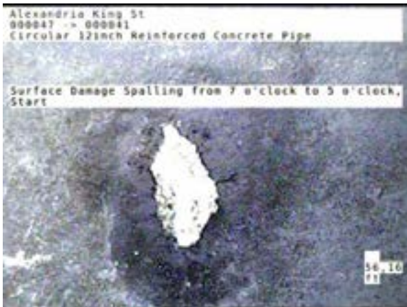
5, 00:04:05, 56.17ft Surface Damage Spalling from 7 o'clock to 5 o'clock, Start
