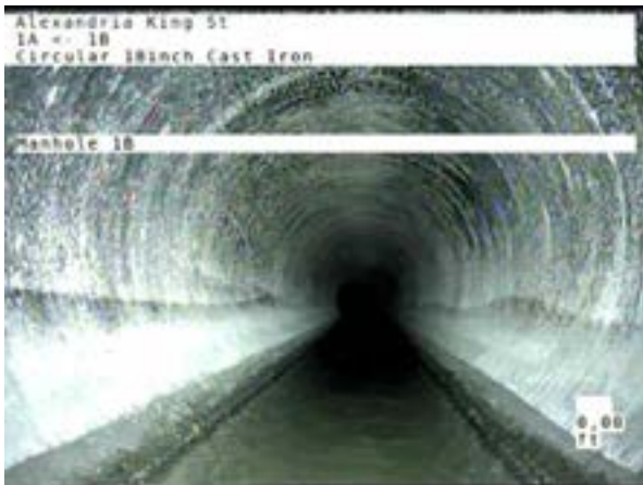
1, 00:00:00, 0.00ft Manhole / 1B
