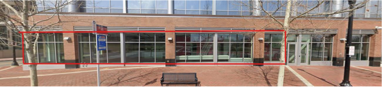
Figure 2- Window sign placement along East Glebe Road
