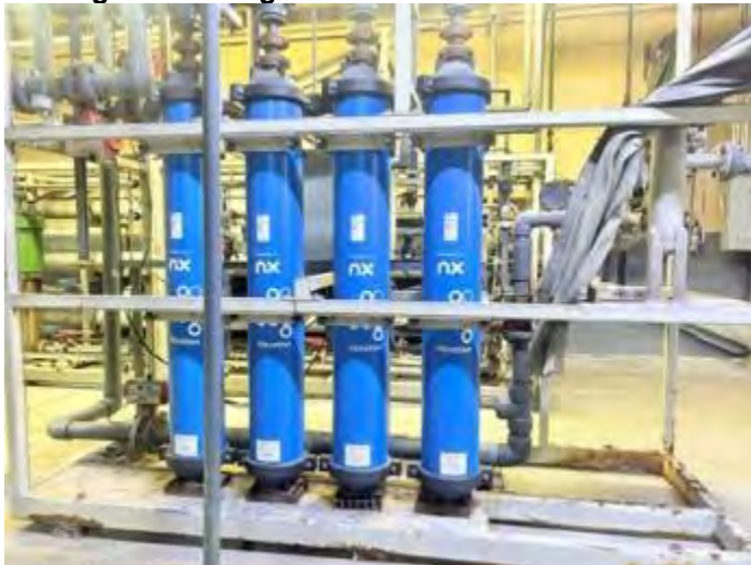
Figure 9: Filtration tanks for Reverse Osmosis System
