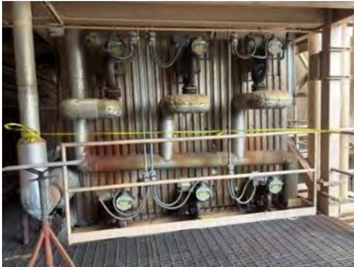
Figure 13: Boiler No. 2 Economizer Rotary Sootblowers
