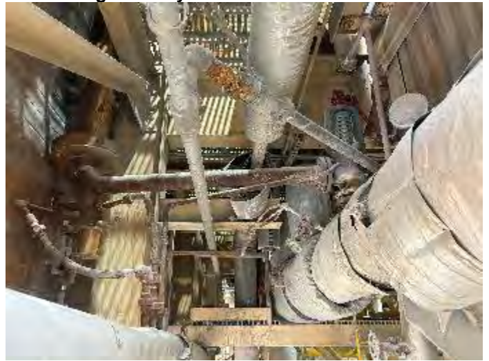
Figure 16: Minor leak on Boiler No. 1 external piping has been repaired – Resolved Deficiency
