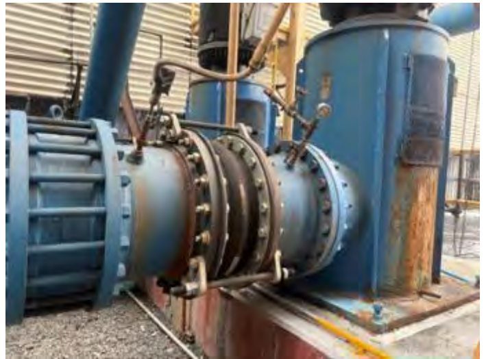
Figure 2: Circulating Water Pump housing is corroded
