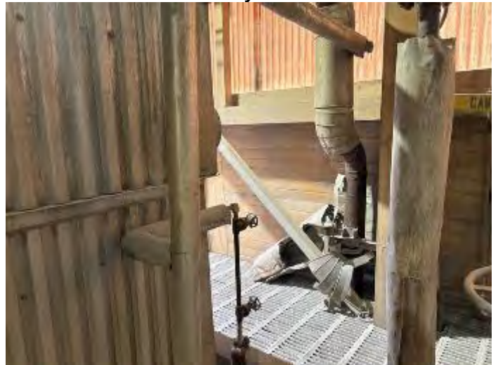
Figure 22: External Tube Leak on Boiler No. 2 right wall repaired
