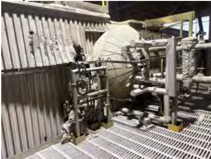
Figure 21: Insulation and lagging damaged around Boiler No. 3 Steam Drum
