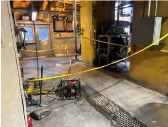
Figure 7: Temporary pump in service for trench drainage to Cooling Tower basin
