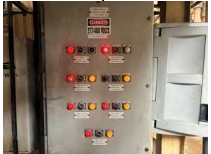
Figure 28: Unit 1 baghouse hopper heaters on and in the manual position
