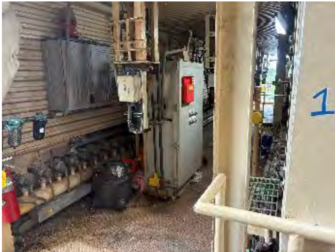
Figure 27: Debris and flyash covering decking inside Baghouse No. 1 Compartment Aisle
