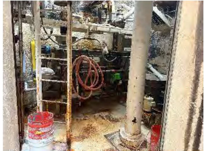
Figure 26: Unit 1 lower lime silo floor with significant corrosion – New Deficiency
