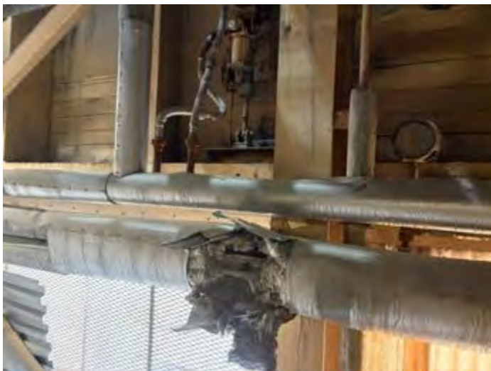
Figure 17: Steam leak repaired on west side of Boiler No. 2 – Resolved Deficiency
