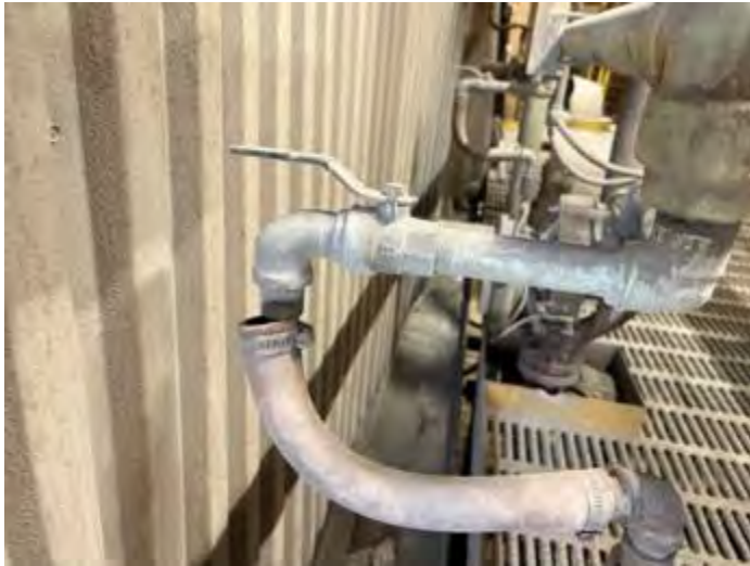
Figure 19: Seal air disconnected on Boiler No. 3 Rotary Sootblower G9-B09
