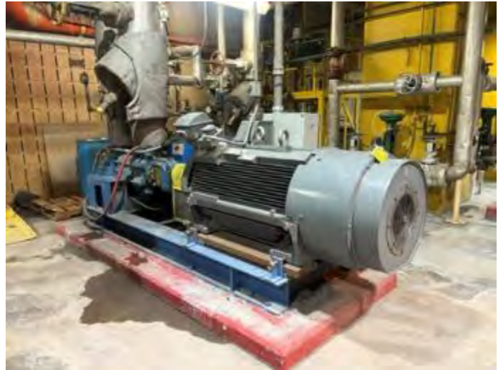
Figure 8: New Circulation Water pump installed
