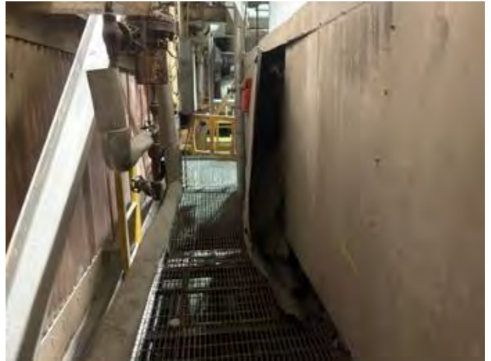
Figure 14: Boiler No. 2 lagging detached and obstructing walkway
