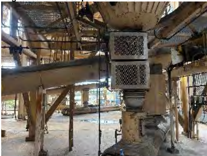
Figure 29: Unit 2 fly ash double dump valves operating properly
