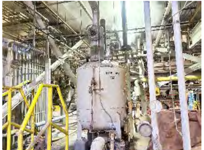
Figure 10: Blow down tank
