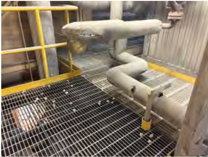
Figure 15: Refractory damaged around Rotary Sootblower G9B-11 on Boiler No. 1
