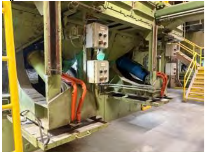
Figure 12: Boiler No. 1 new Run 2 grate drive cylinder
