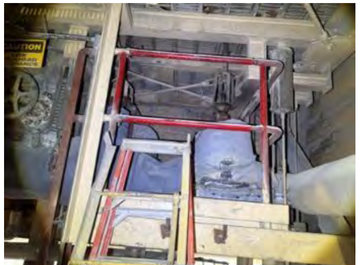
Figure 18: Insulation added around steam isolation valve on Boiler No. 3. – Resolved Deficiency
