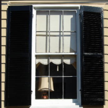
^ 6/6 FEDERAL / GREEK REVIVAL
