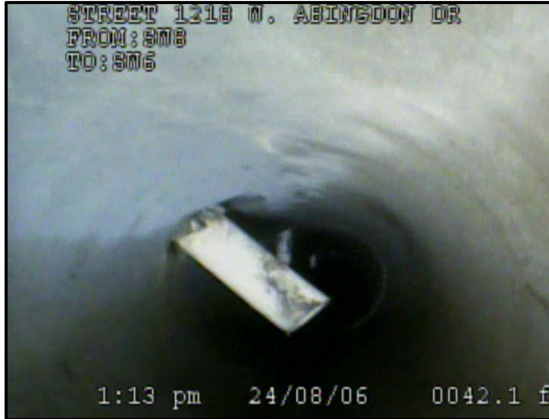
Image 1. Lateral Connection in storm sewer
