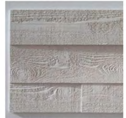
BOARD-FORMED CONCRETE PANEL TO REFERENCE HISTORIC CRIBBING
