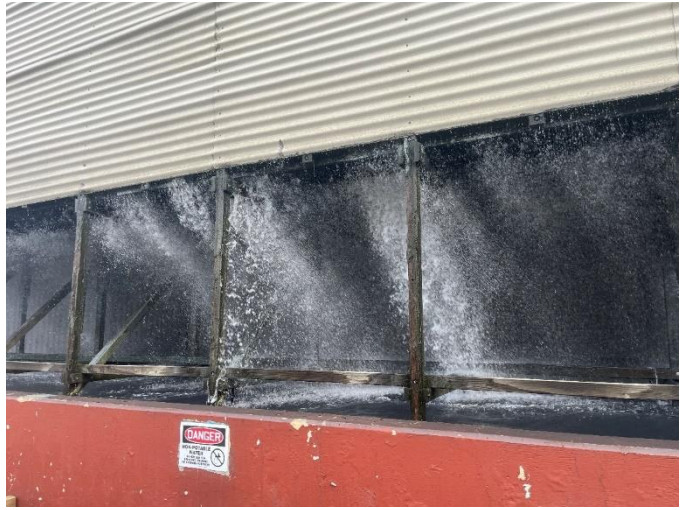
Figure 2: Cooling water tower appears to have some uneven flows. Deficiency Number 10.
