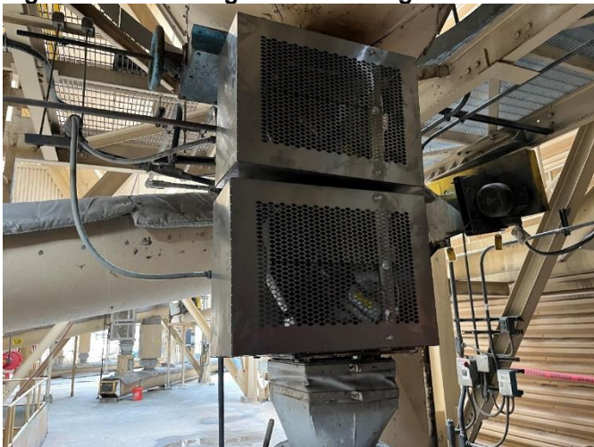
Figure 23: New safety cages installed around dump valves
