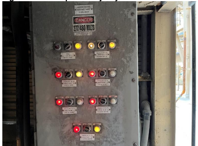
Figure 24: Hopper Heater Controls set to manual with Low Temperature Indicators on
