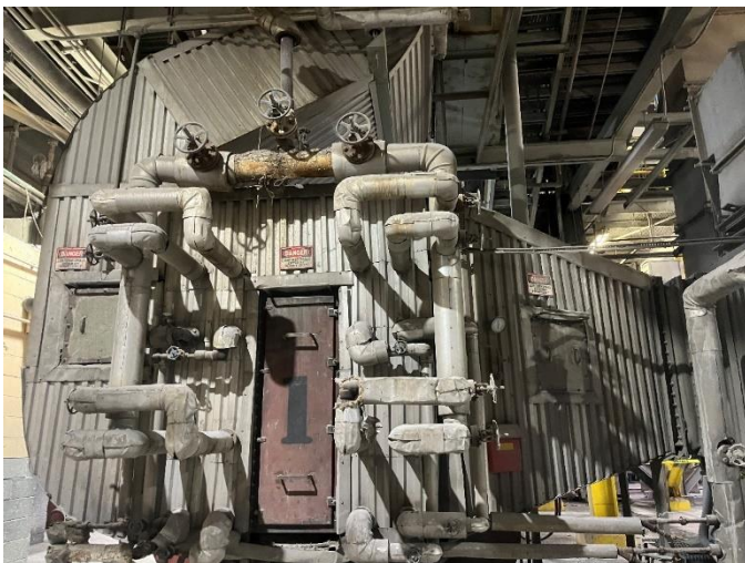
Figure 11: Unit 1 forced draft fan and under fire air coils
