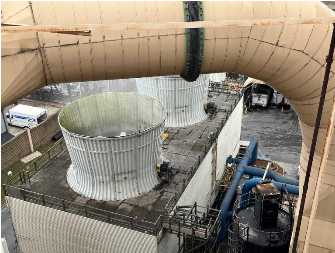
Figure 19: Cooling Tower Deck cleared of material
