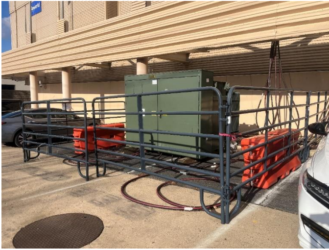
Figure 1: Back-up transformer on-site
