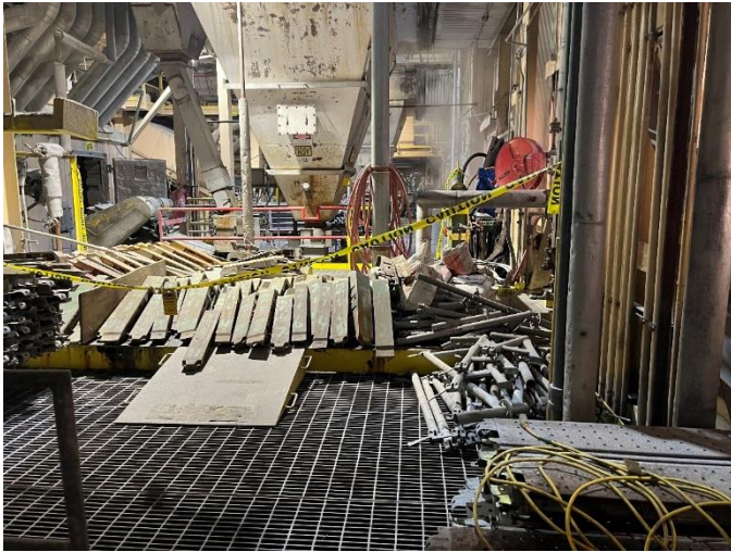
Figure 13: New grate bars prior to installation during Unit 3 Major Outage
