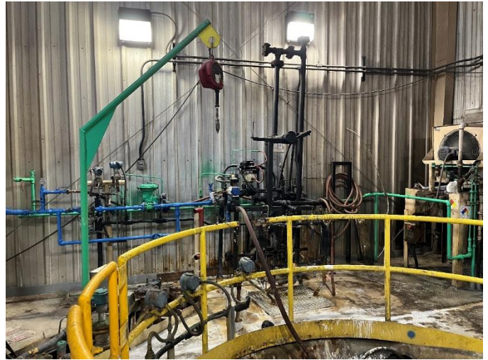
Figure 20: Recently painted Lime Slurry Pipes in SDA Penthouse No. 1
