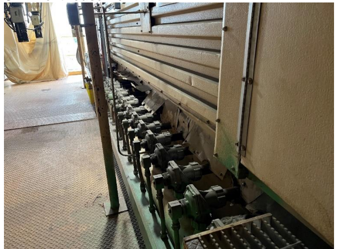
Figure 22: Unit 1 pulse air jet system
