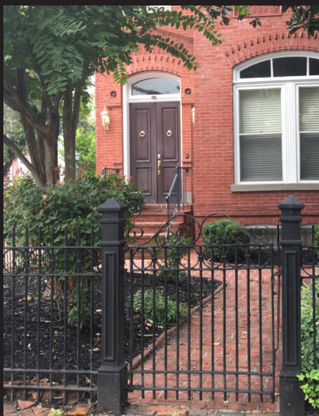
A wrought-iron fence on a Victorian-style residence.
