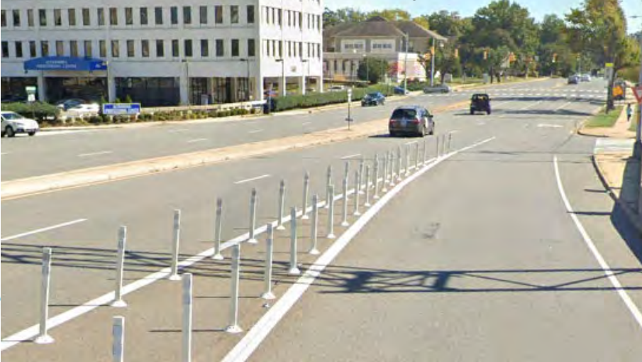
Prevent illegal turns with flexiposts - Example on Seminary Road
