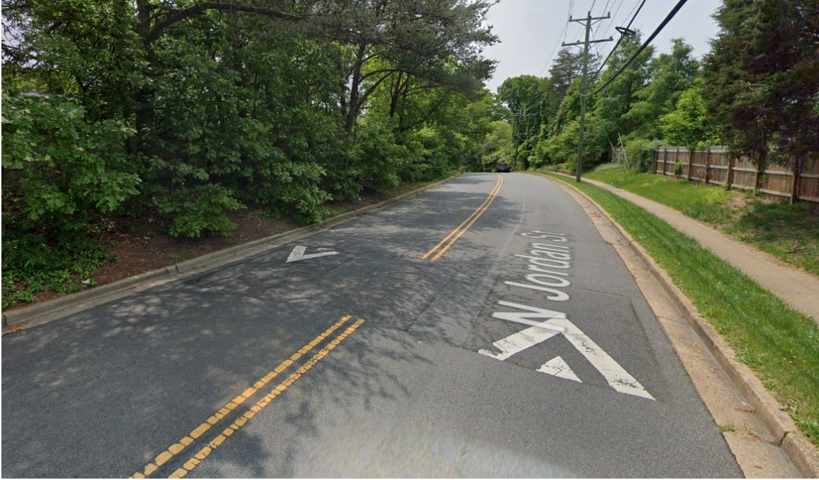
Speed Cushions along North Jordan Street, Alexandria, VA
