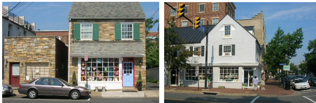
Figure 6: Old Town businesses must work with multiple property owners and retrofit small historic buildings for modern merchandising to meet consumer demands.
