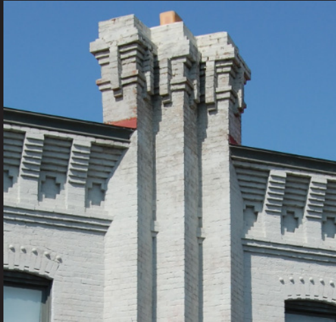
The corbelled brick chimney is a character defining feature of this Queen Anne style residence.
