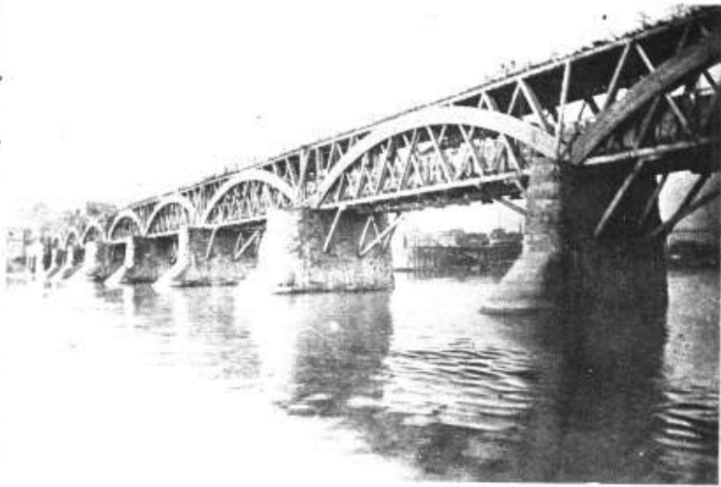
TWO-TIERED AQUEDUCT BRIDGE
