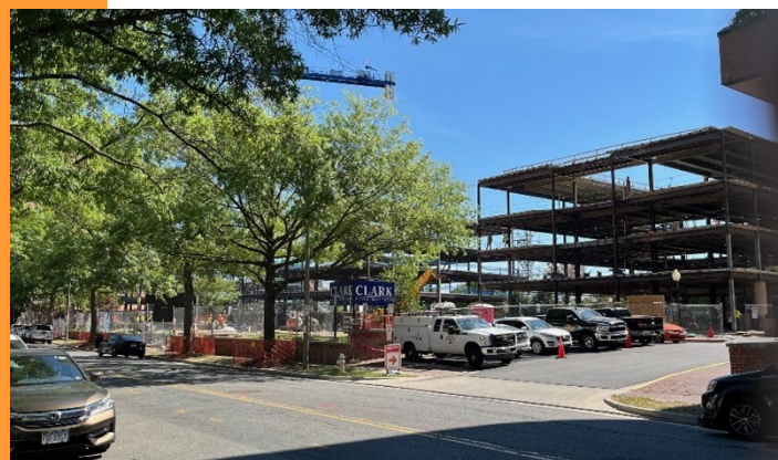
Site under construction, summer 2024
