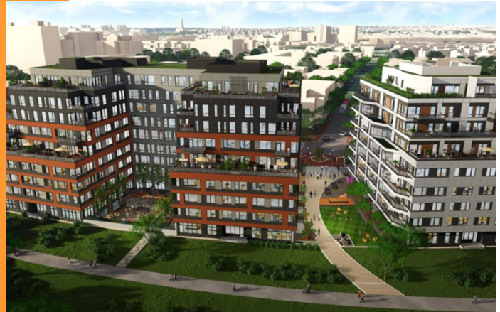
View of entire site from east elevation
