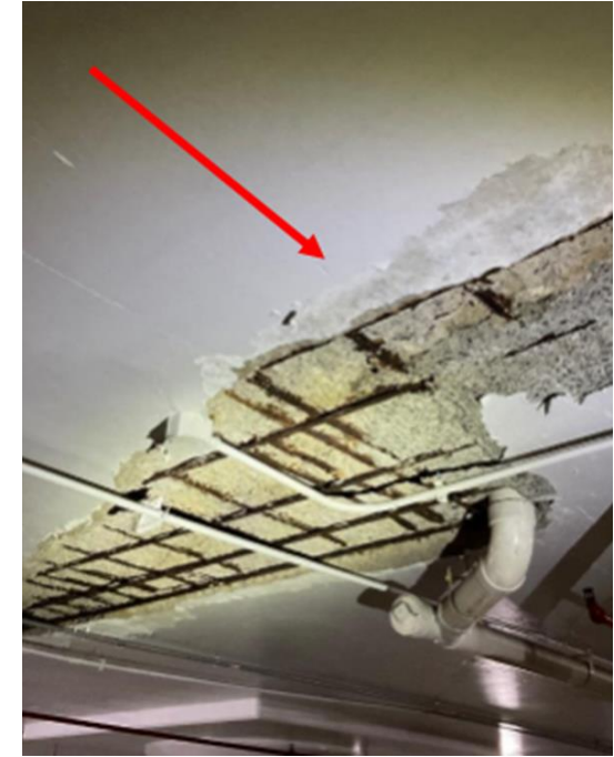
Exposed structure at parking garage
