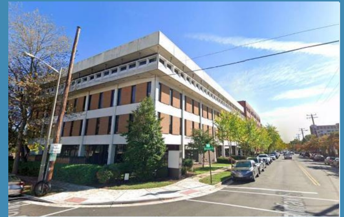
Then: Waterfront Center office buildings
