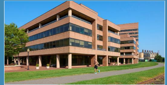
Existing: TransPotomac Plaza Office Buildings
