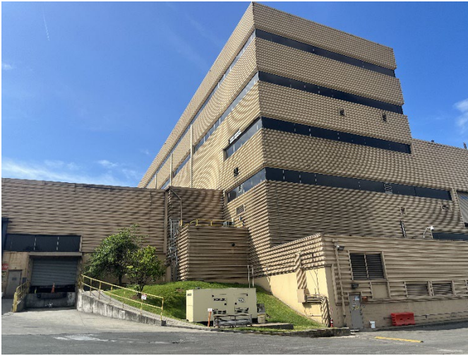
Figure 1: North Side Of Building Beginning To Look Dirty.
