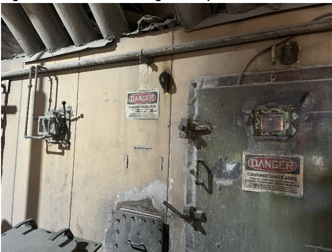
Figure 11: View Ports All Boilers Covered And Repaired.
