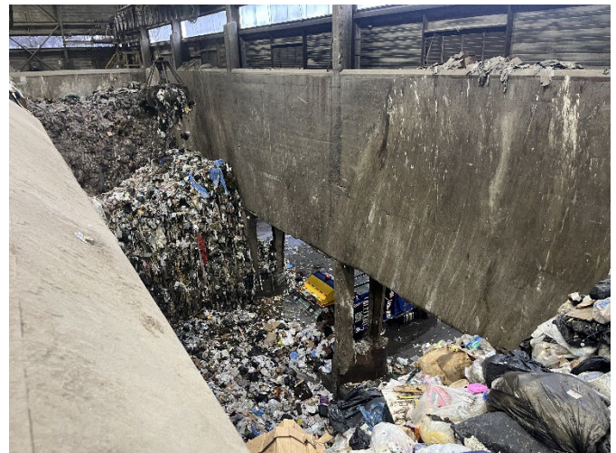
Figure 30: Refuse Pit Level.
