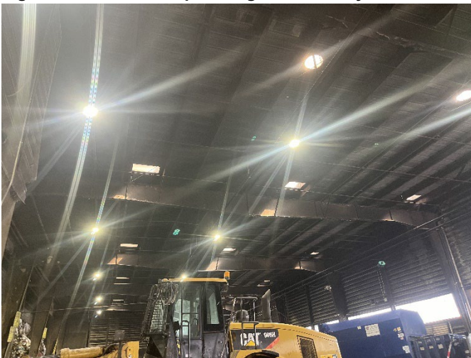
Figure 5: New LED Lights Installed Over Tipping Hall.
