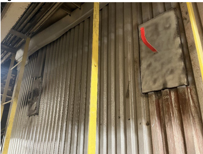
Figure 17: Boiler No. 3 Viewport Capped For Repair. Closed On Punch List.
