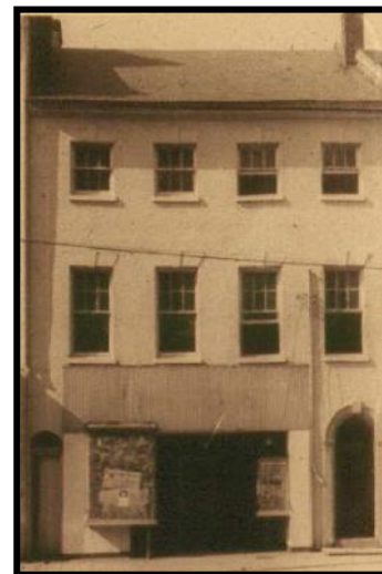
518-520 King St., 1967 before demolition
