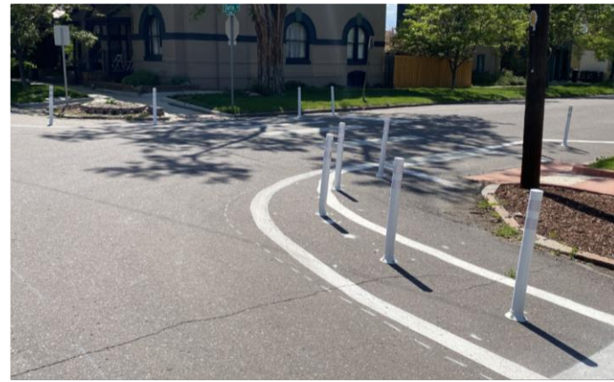
Curb Radii Tightening
