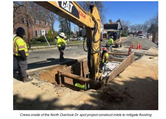
The City contractor has started work to improve drainage and provide flood relief near the intersection of North Overlook Drive and South Overlook Drive. The project will increase inlet capture and runoff conveyance capacity to mitigate flooding for residents in the area. Traffic is being managed near the project site and drivers can expect some delays.
