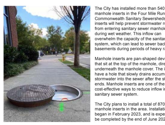
manhole inserts in the Four Mile Run and Commonwealth Sanitary Sewersheds. These inserts will help prevent stormwater runoff from entering sanitary sewer manholes during wet weather. This inflow can overwhelm the capacity of the sanitary sewer system, which can lead to sewer backups in basements during periods of heavy rainfall.
