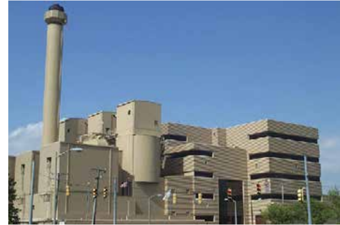
COVANTA Alexandria/Arlington Waste-To-Energy Facility
