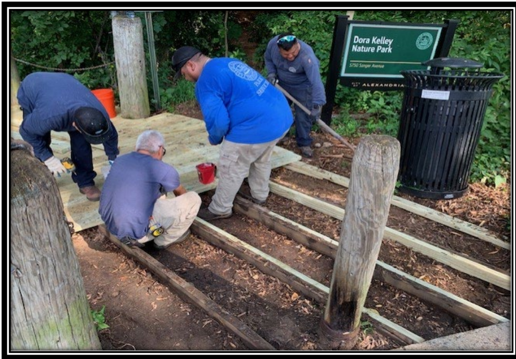
Restoration of the Boardwalk/Bridge at Holmes Run/Dora Kelley Trail
