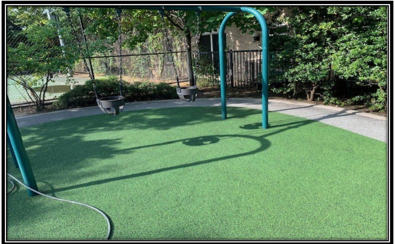
Playground After Power Washing
