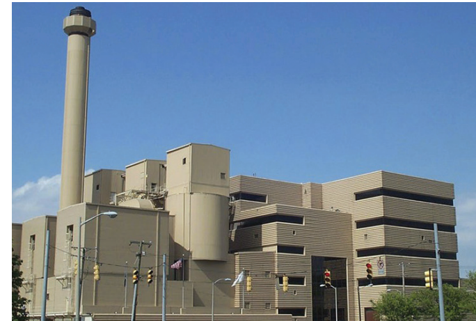
COVANTA Alexandria/Arlington Waste-To-Energy Facility
