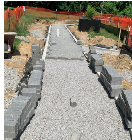
Permeable pavement BMP under construction at the Fort Ward picnic shelter pathway
