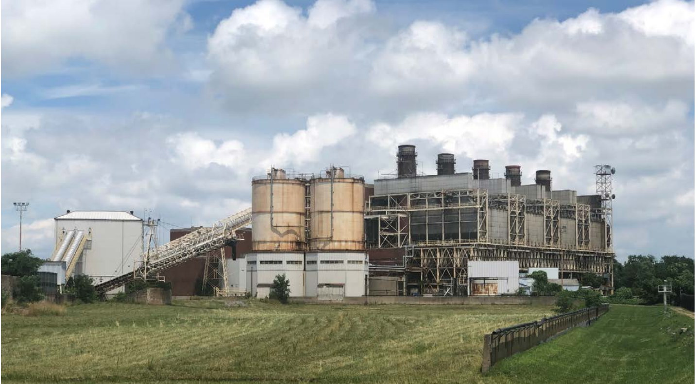
Figure 1. Former PRGS Coal Plant
