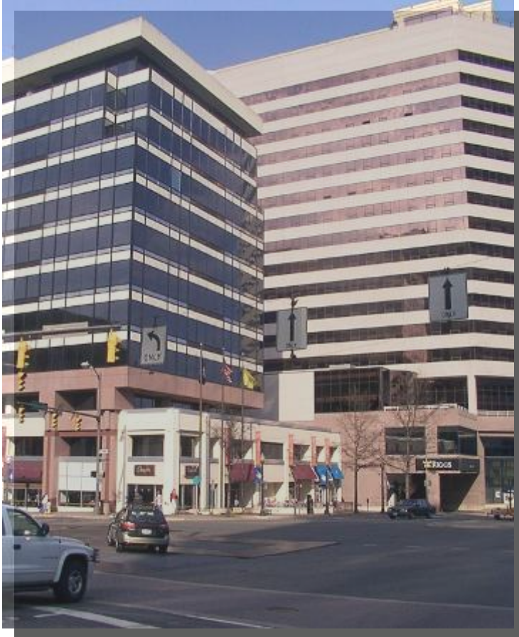
Inappropriate Horizontal Banding
