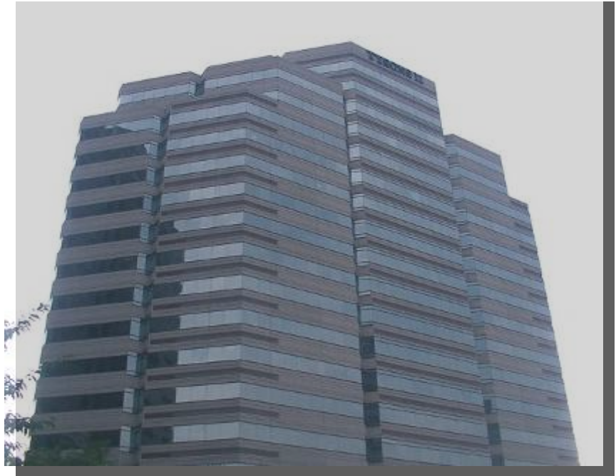
Inappropriate Horizontal Banding
