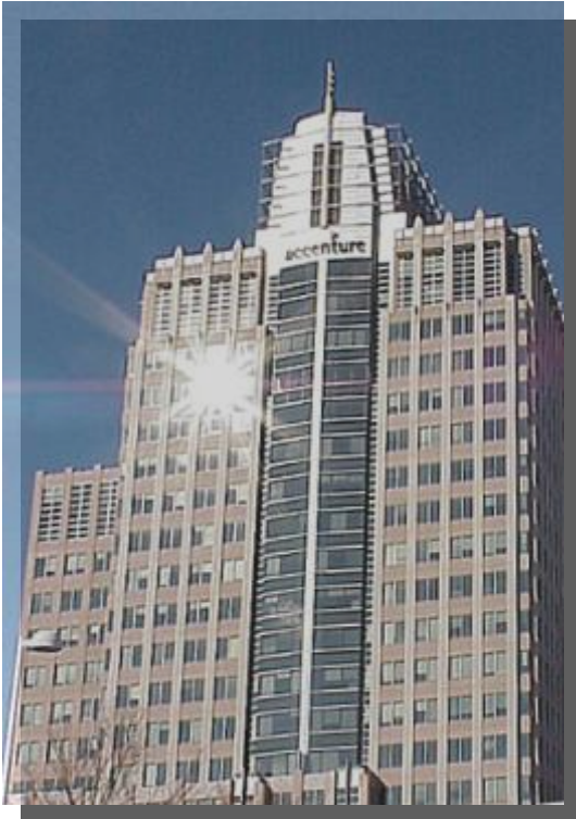
Distinctive Tower Top
