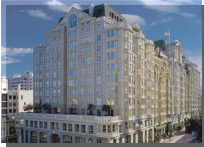
Tower set back from the streetwall
