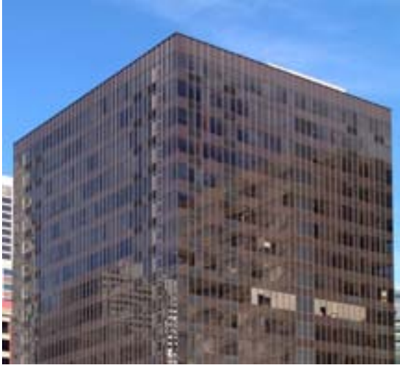
Inappropriate all glass facade
