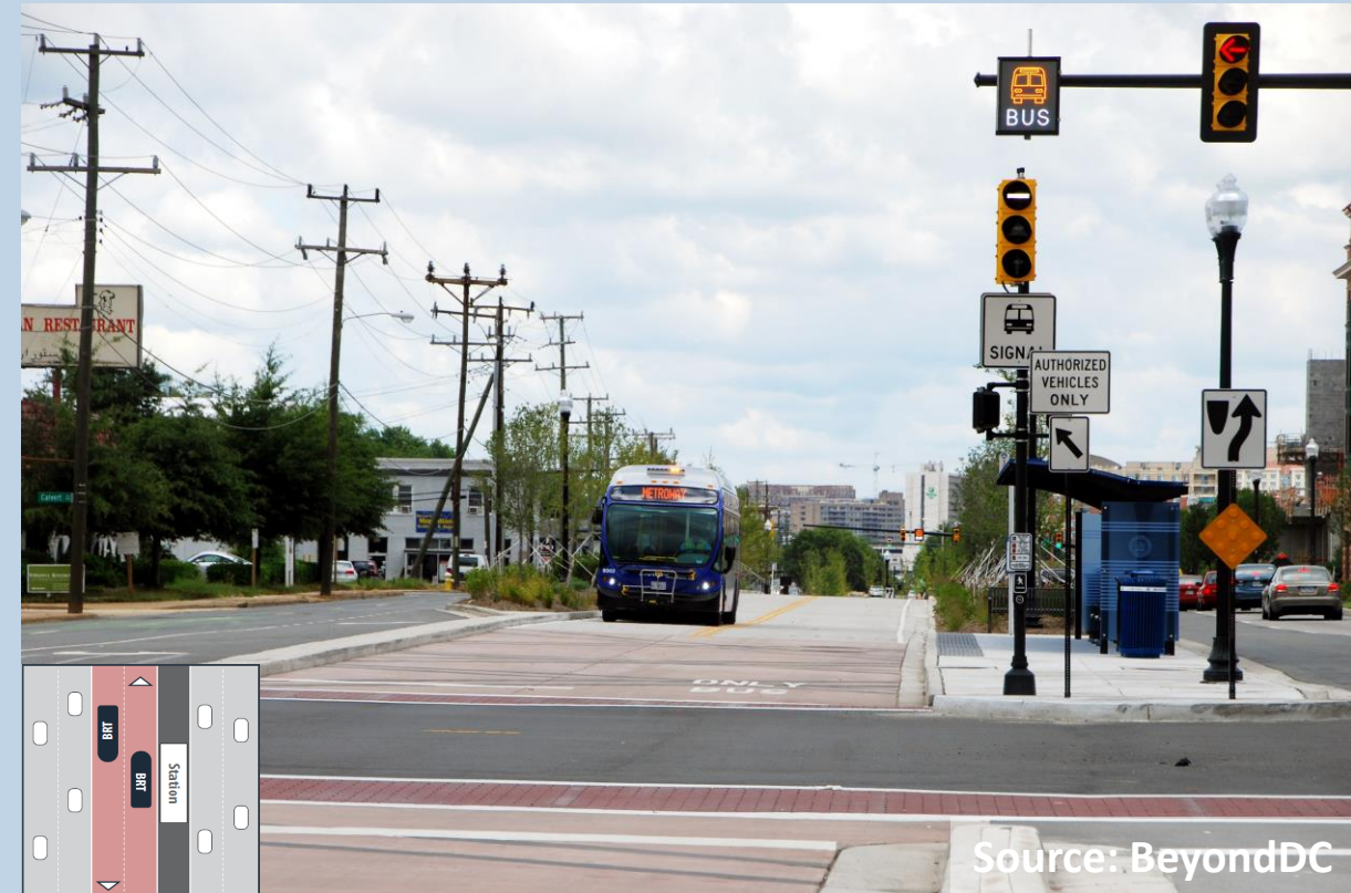
Metroway BRT, Alexandria, VA
