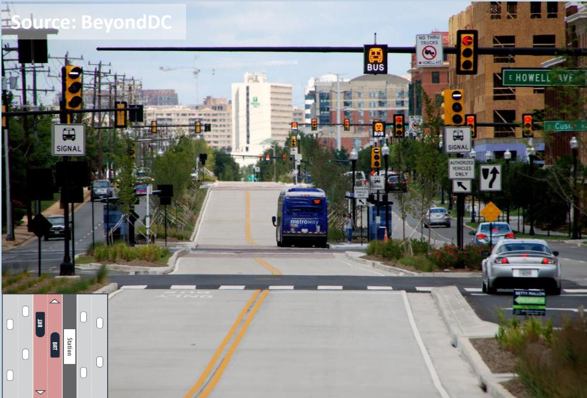
Metroway BRT, Alexandria, VA
